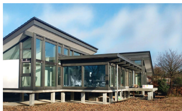
Figure 10. An example of a building with elevated ground floor slab
