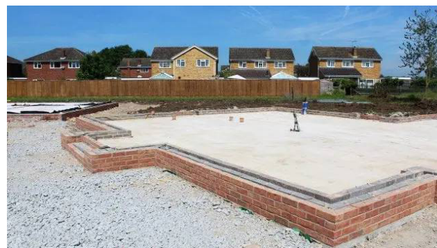
Figure 9. An example of a building with elevated plinth level
