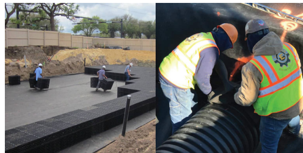
Figure 28. Storm water tank management systems (Ferguson, 2023)
